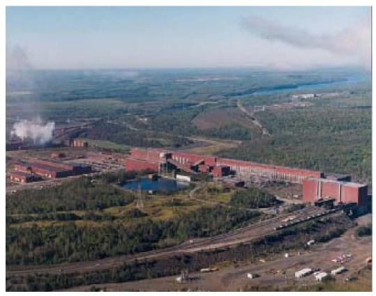
The whole plant is reported to have cost approximately US\$350 million in the 1950s. It can best be described as being 1950s American engineering at its best. The photograph above on Page 13 shows an aerial view of the plant – the ore cars arrive at the primary crusher to the right of the photograph. Crushed ore is then fed up the conveyor (center) and then feeds a bank of some 34 mill circuits in the long building that stretches across the picture.
